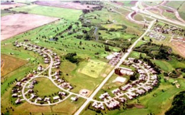
Clustered development that maximizes open space for both human and wildlife use. Note the building setback from the river.
